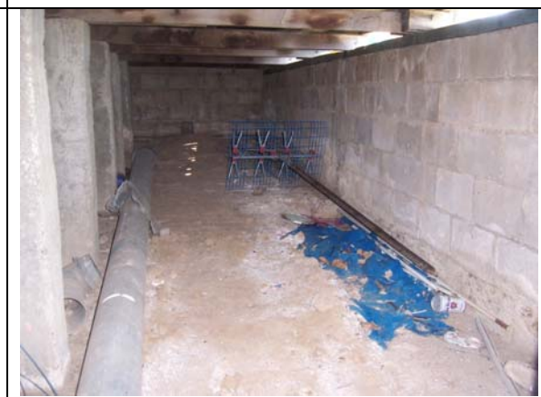
Figure 8 - Concrete pier, blockworks & foundation under veranda
