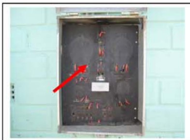
Photograph 5: Meter box backing sheet (Sample No. 4447 – V 3 )
