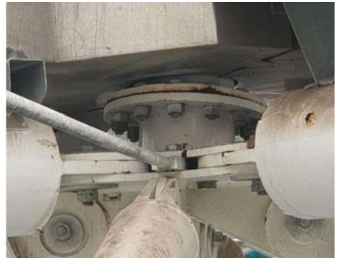
Image 3: Identification of Corrosion
