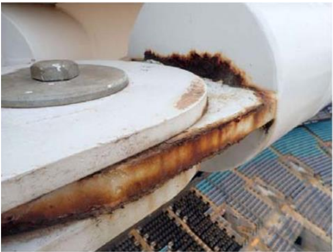
Image 3: Identification of Corrosion
