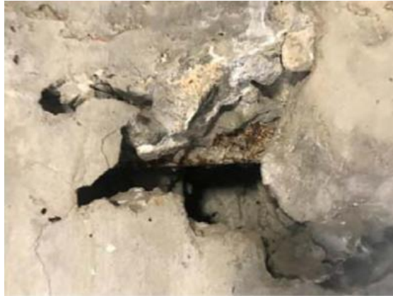
Image 4: Partially exposed reinforcing bar depicted in report BCRC N0734 (06/02/2020)
