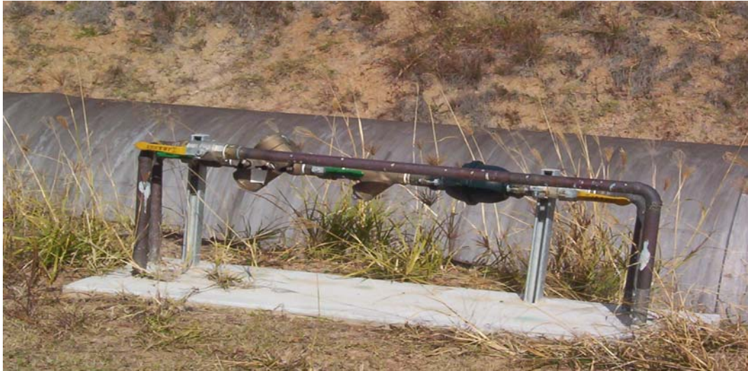
Customer off-take pipeline and meter
