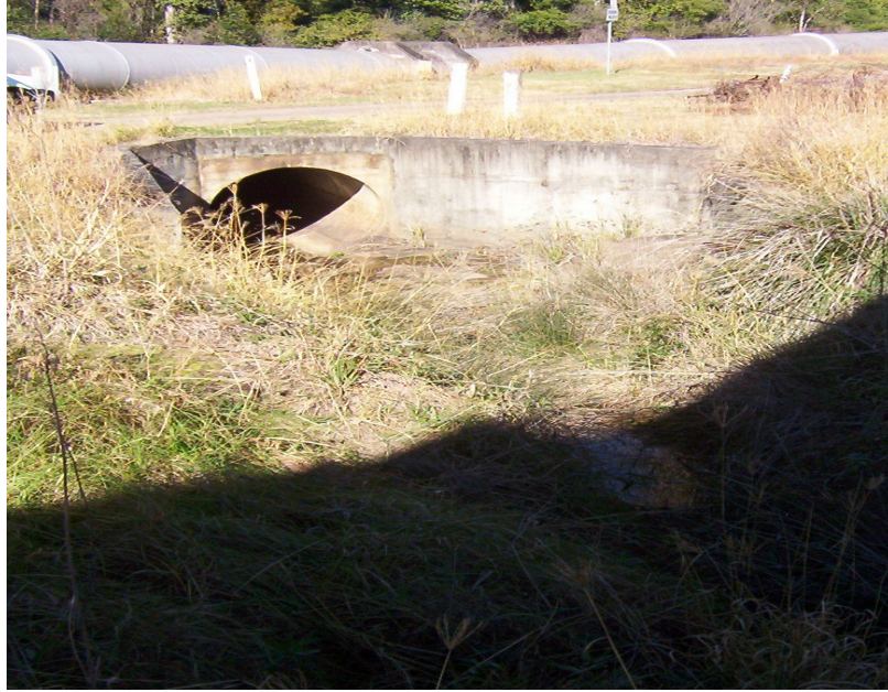
Creek with headwall & sidewall
