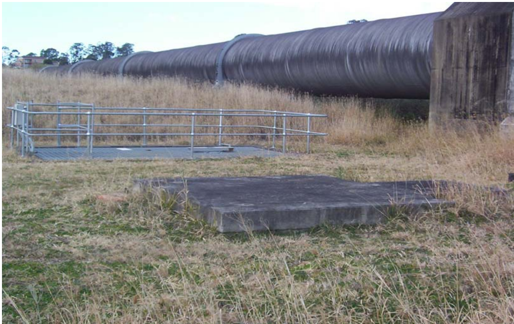
Valve chamber in ground
