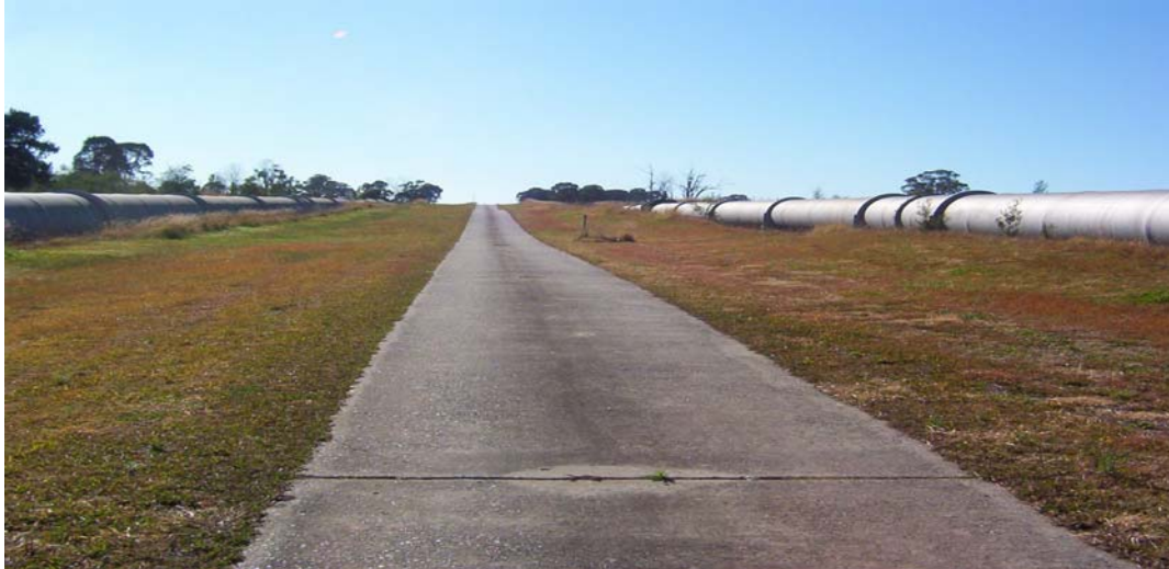
Typical SCA concrete roadway (level with surrounding ground level)
