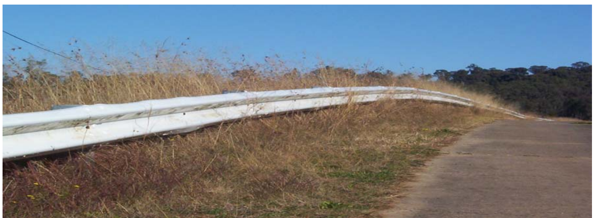
Armco railing
