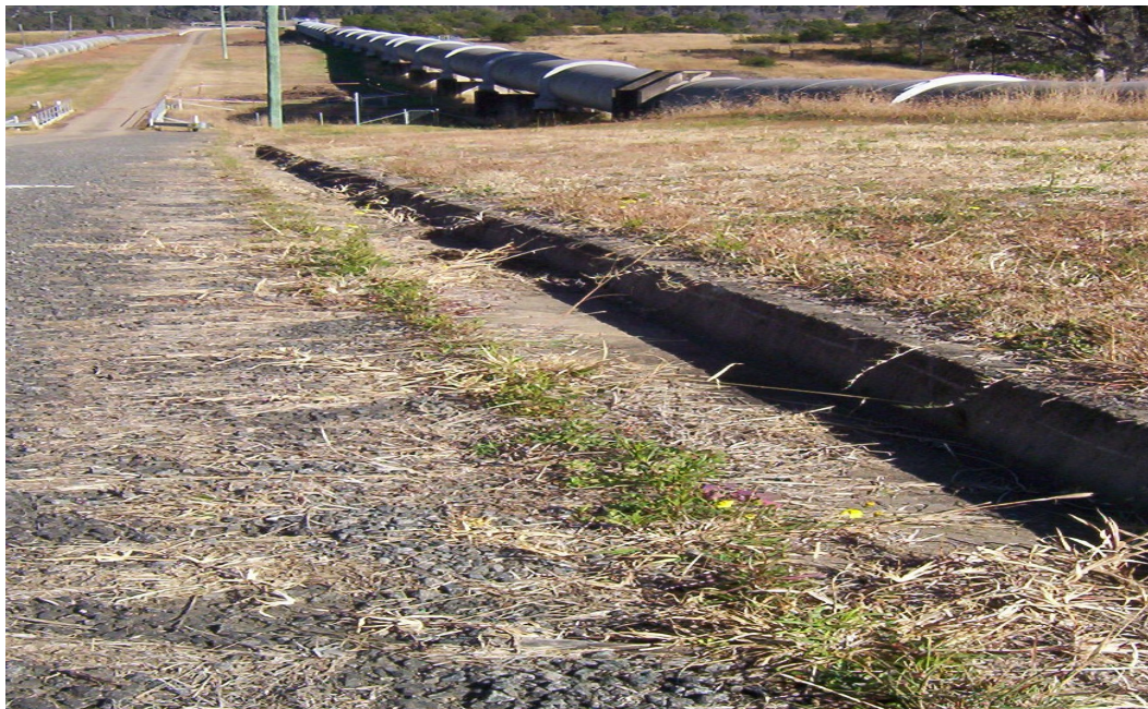
Roadway with kerbed gutter (road is below surrounding ground level)
