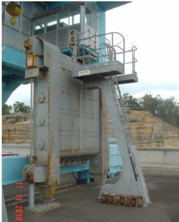
Figure 1: 2100mm Emergency Gate at Warragamba Dam
