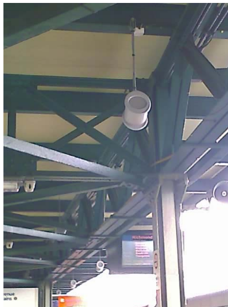
Figure 4 Example of interference of loudspeaker locations by roofing trusses
