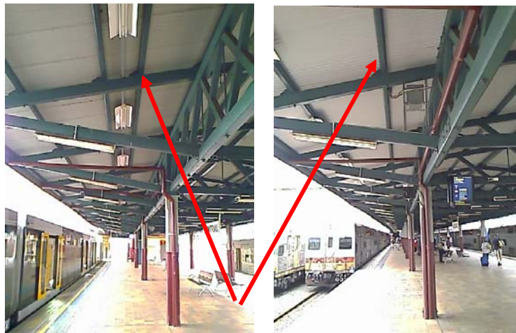
Figure 3 Fixing location for loudspeakers on Platforms 4 to 15.
