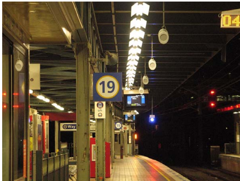
Figure 2 CS6 loudspeakers as implemented in Proof of Concept project
